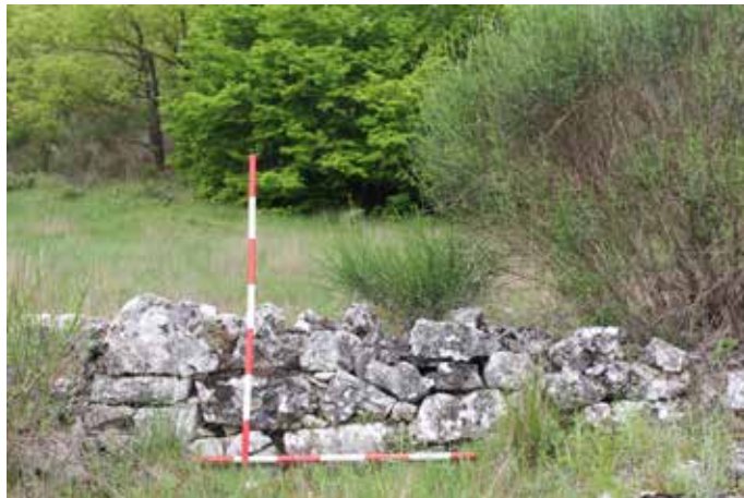
Remains of a fortification wall in Il Monte - Santo Spirito (Grumento Nova)
