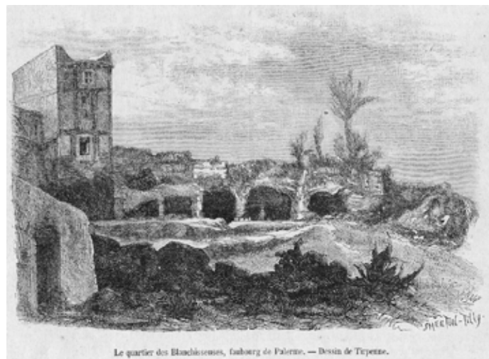
Fig.1: An engraving published by the French Journal “Le Magasin Pittoresque” in 1874. It illustrates a building in Palermo located in the unknown “Laundrywomen district”. Note the extraordinary similarity to an ancient theatre.
